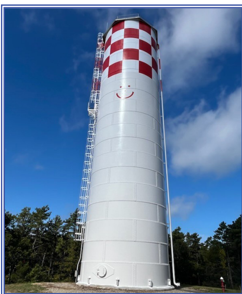
Mary Dunn 1 Water Storage Tank rehabilitation completed
